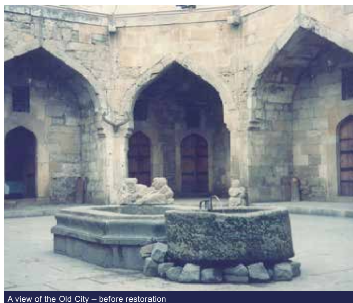
A view of the Old City – before restoration
