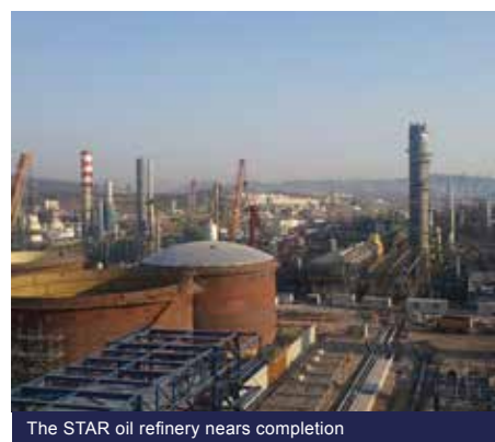
The STAR oil refinery nears completion
